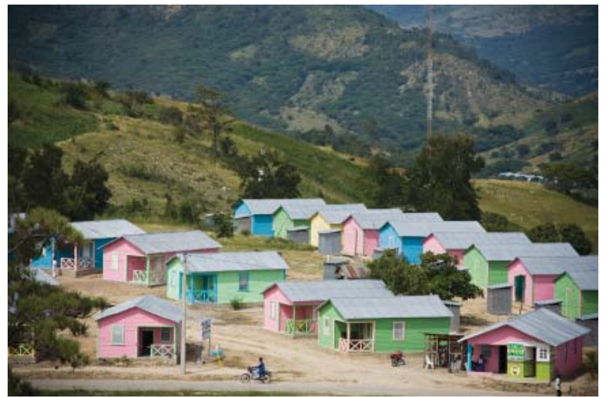
La Siembre Vieja Community Housing project is a rainbow of color in the mountains. FFP has built 60 of these brightly painted homes, along with latrine projects, a water project, and a rural school.
